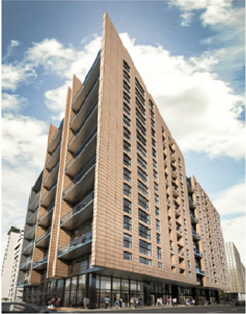
Visual of the proposed development – corner of Cheetham Hill Road and Lord Street
